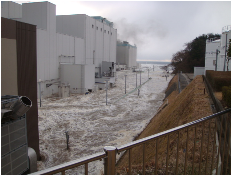
Fukushima I nuclear power plant, Japan 11 March 2011
